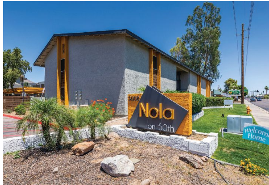
Constructed in 1979, Nola on 50th features 12 buildings on 5.6 acres of land and offers a mix of studios, one- and two-bedroom units.
